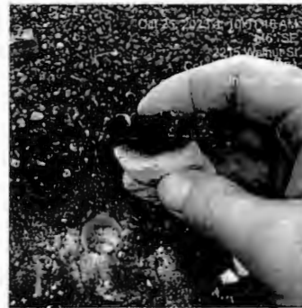
Core Cut: 6" Total XPS and Lightweight Concrete with 2 ply flood and gravel.
